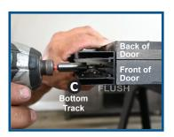
Make sure the Bottom Track is **flush** with the front of the door and in the correct location before drilling. Pre-drill holes into the door for the supplied screws. Then use the provided screws and attach the Bottom Track to the bottom of the Door Slab.
