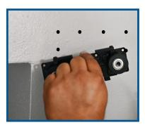
Next, pre-drill all (6) pencil marks. Use supplied screws & anchors to attach Wall Mount. **Do Not Over-Tighten.**
